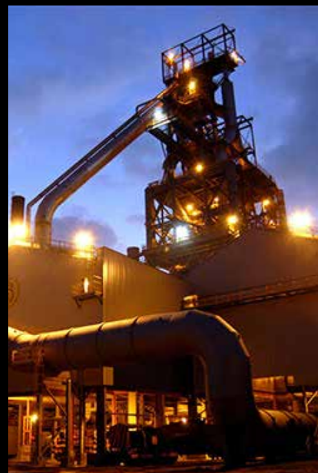
Port Talbot Steelworks. Wikipedia. en.wikipedia.org/wiki/Port_Talbot_Steelworks
